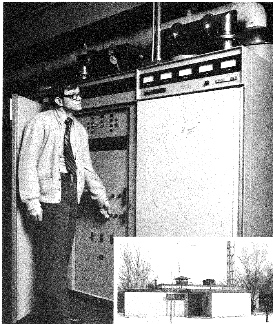
GATES BT-55U IMPROVES SIGNAL, COLOR—Don Clausen, WRAU-TV Chief Engineer, reports that the new Gates BT-55U kW UHF transmitter was the only one which met all the station's requirements for signal strength, color fidelity, and installation compactness. The inset photo shows the trim, functional transmitter building and part of WRAU-TV's 656-foot antenna tower.
